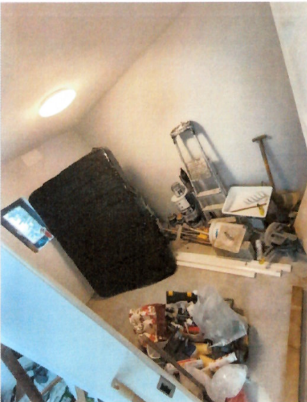
Fig. 7D: The interior of the structure (unchanged from the site visit conducted by the WCC Enforcement Officer)
