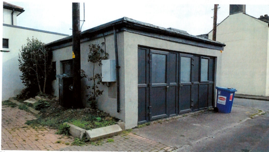
Fig. 5: The location and appearance of the existing structure within St. Kevin's Square – Client photo 2025
