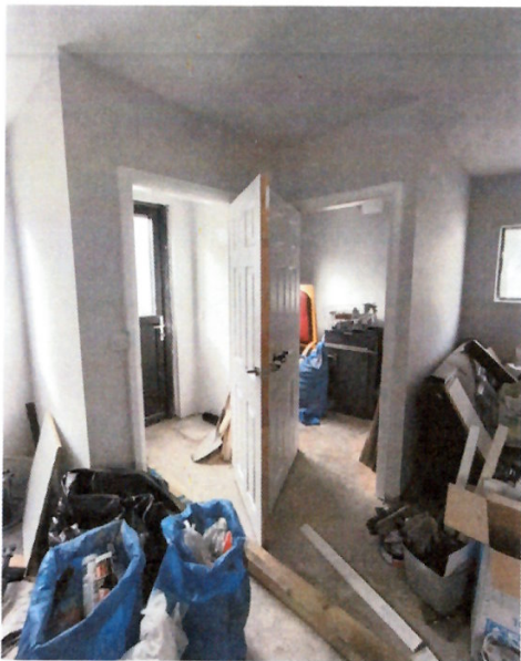
Fig. 7B: The interior of the structure (unchanged from the site visit conducted by the WCC Enforcement Officer)
