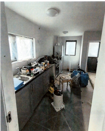
Fig. 7E: The interior of the structure (unchanged from the site visit conducted by the WCC Enforcement Officer)
